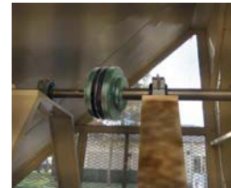
Cooler Jack Shaft with Sure-Flex® Plus Coupling
