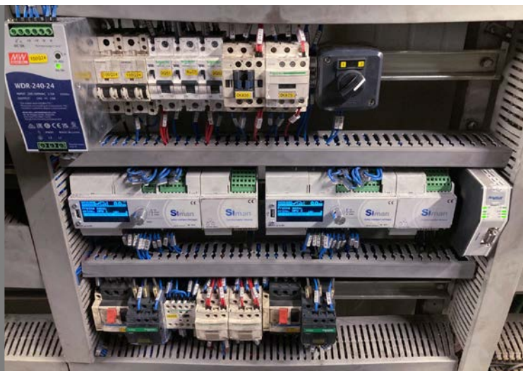
Revamping / 130T ITALGRU ITON Seine crane with SIMAN and SIMAN-CM modules and Interface for monitoring
