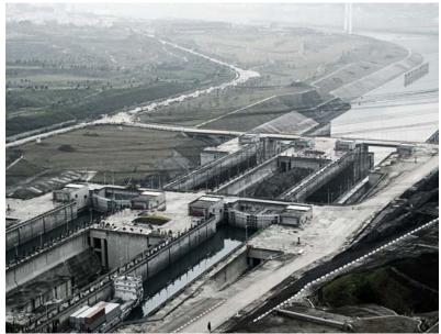
The dam's ship lift will shorten the time taken for ships to pass the dam from three hours to one. Svendborg Brakes became the chosen provider of among others 32 brakes acting as parking brakes, respectively security brakes for the electrical drive.
