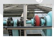
Dura-Flex couplings withstand harsh conditions in wastewater facilities.
