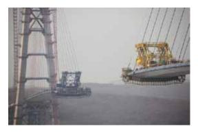
The central span of the bridge is made up of 103 panels, each 12m long, 26m wide, and weighing 300 tons.
