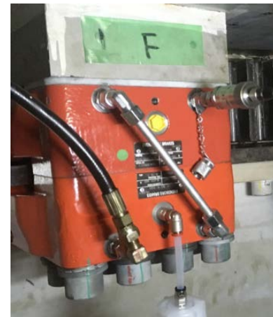
Fig 2: Assembly inside Nacelle after retrofit
