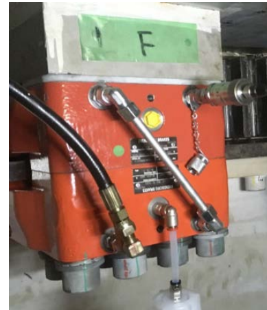
Fig 2: Assembly inside Nacelle after retrofit
