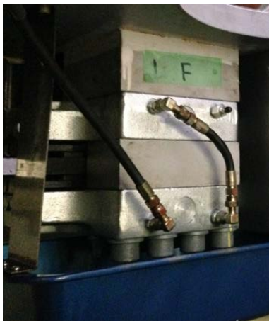
Fig 1: Assembly inside Nacelle before retrofit.
