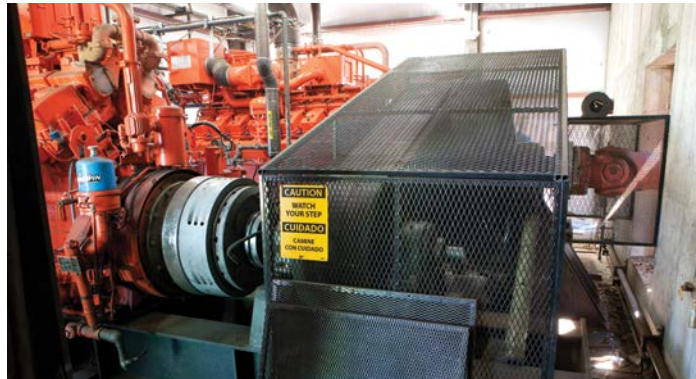
The photo above shows a Wichita clutch (left), TB Wood's sheaves and belts (center, under grated guards), and an Ameridrives U-Joint (far right).
