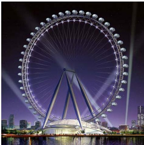
There are 48 underhung cabins on the world's tallest Ferris wheel in Beijing, China. Each cabin is equipped with a Warner Electric linear actuator and electromagnetic tooth clutch.
