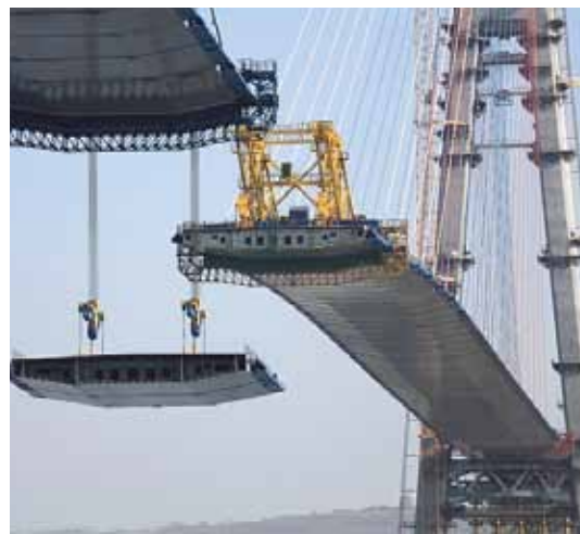
The Mostovik crane lifts 300 ton bridge panels 70m into position.
