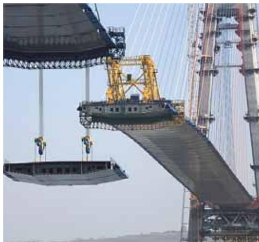
The Mostovik crane lifts 300 ton bridge panels 70m into position.
