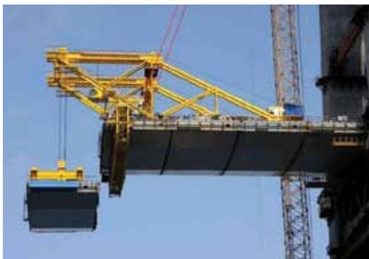
A custom-designed Mostovik derrick crane was installed on the bridge center span deck, cantilevered over the nose and facing toward the strait.
