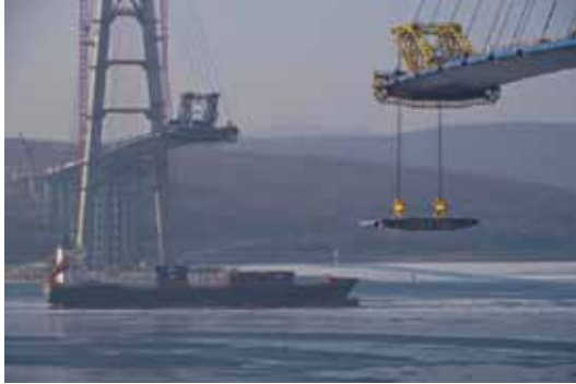
Bridge panels are delivered by barges, which are positioned under the installation using GLONASS, a Russian global satellite navigation system.
