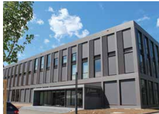
In addition to the state-of-the-art production facilities, the new, 30,000m 2 facility includes a new conference centre and open plan offices.
