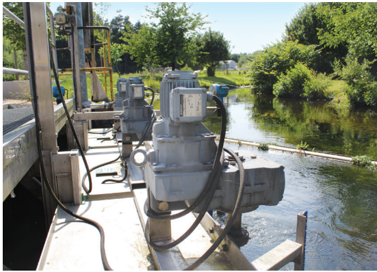
For many years, nrw Anlagentechnik has specified Bauer gear motors to operate its vertical brush systems.
