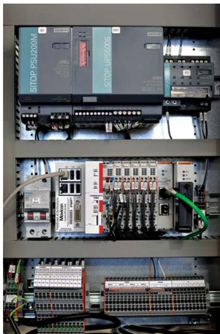
SOBO iQ units have three-state digital modulation – never used in a braking system before. Each controller can accommodate up to 4 HPUs with defined torque sharing. Other features include full BUS-based communication with the master control system.
