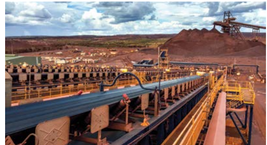
Roy Hill iron ore mining, rail and port project in the Pilbara, West Australia.
