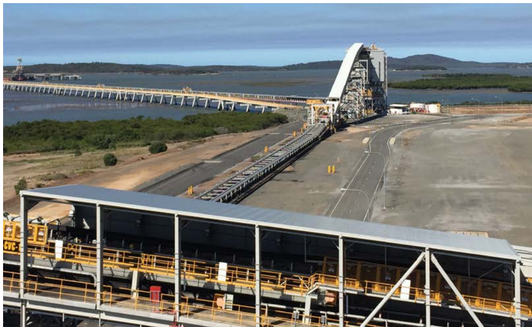
Wiggins Island Coal Export Terminal (WICET) in Queensland, Australia.
