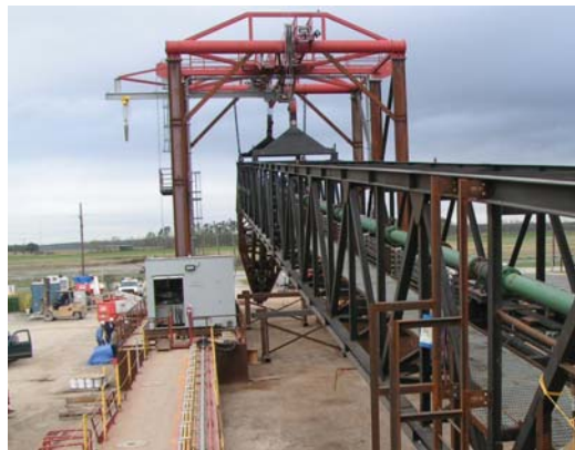
After fabrication and testing, the Marlin mining dredge was disassembled and loaded onto 23 tractor trailers for transport to the Florida "pond" where it will operate until the middle of the 21st century.
