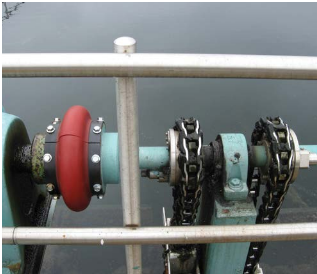
Couplings have to withstand the harsh conditions of wastewater facilities, including water and chemicals, high shock loads, constant operations, extreme temperatures and UV radiation.
