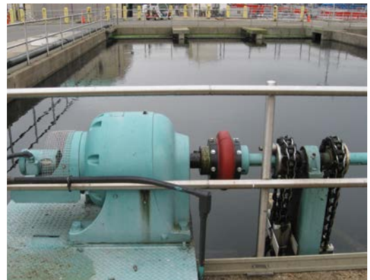
TB Wood's Dura-Flex couplings employ a light-weight element that absorbs shock loading and torsional vibration. A specially formulated elastomeric material offers superior chemical, dynamic, and weathering properties.
