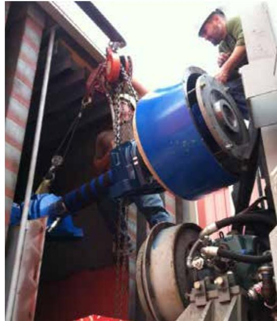
Pre-assembled drive shaft, with Wichita Standard Ventilated Clutch, is lifted into place during final drivetrain installation.
