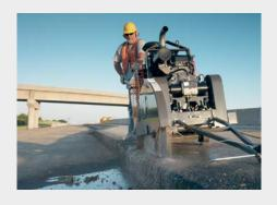
**Problem:** Adding an electric clutch to a concrete saw system adds both convenience and safety to these high demand, but potentially dangerous systems. The application has multiple design challenges. The system must be able to work reliably despite load spikes that can occur when cutting the concrete. High levels of moisture from the cutting coolant could contaminate a clutch with friction material. Lastly, the unit must work in both hot and cold weather situations.
